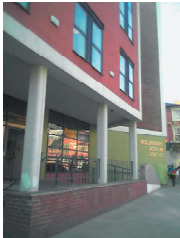
NCVS Building 7 Mansfield Road Nottingham
