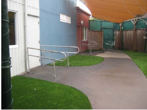
Turf and handrails installed
