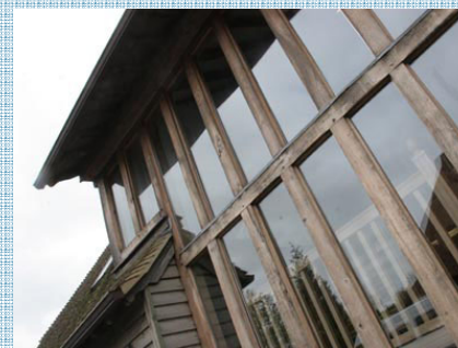
Harvey's Barn, under investigation
